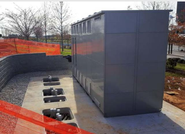
*1475 kVA MV multi secondary mini-substation awaiting charger power modules.*
